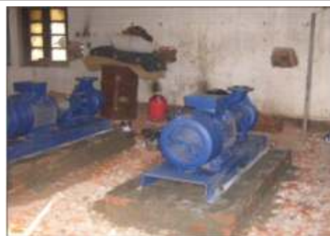
Photo of newly installed pumps with motors in Jaranwala Town
